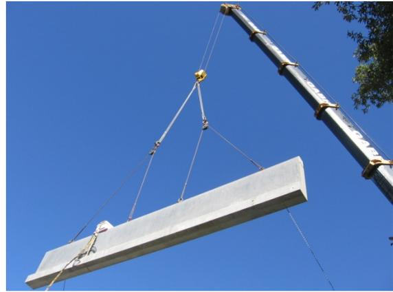
b.) Lifting of Spandrel Beam with DAS Box Attached
