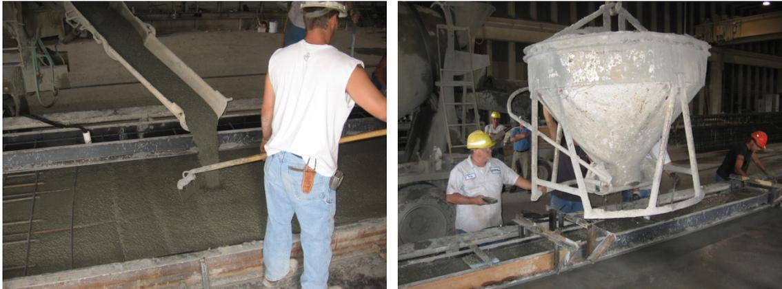
a.) Web Placement with Concrete Truck
