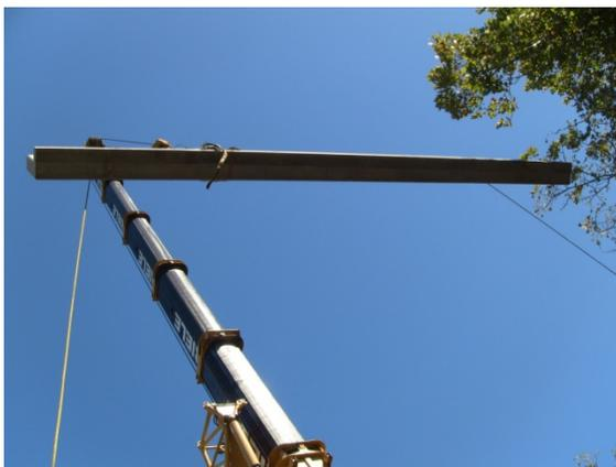
a.) Crane Lifting Instrumented HS-SCC Beam
