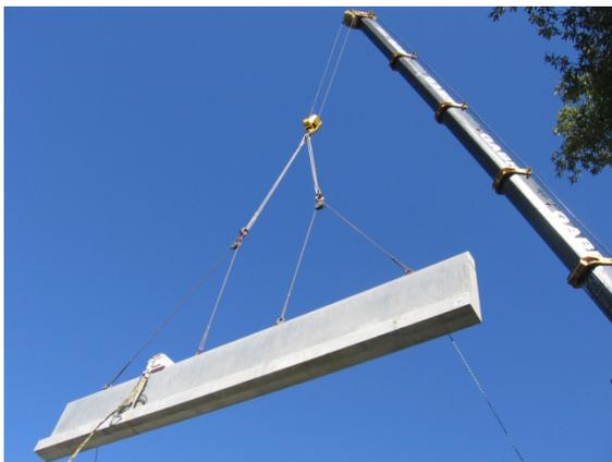
a.) Crane Lifting Instrumented HSC Beam
