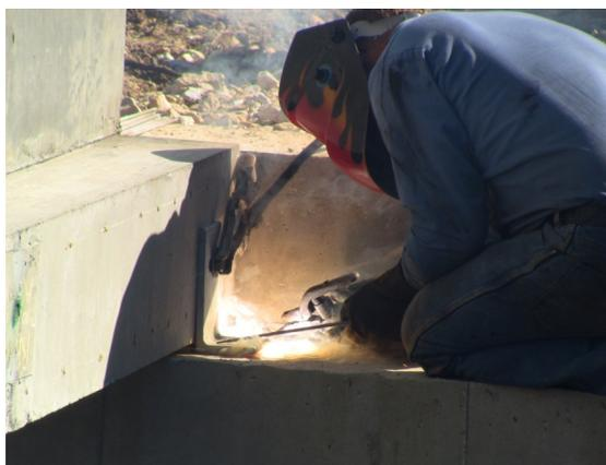
Figure 4.11. HSC Beam Welded to Abutment.
