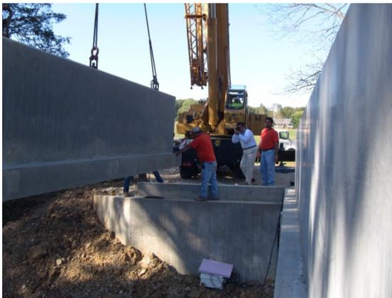
c.) Non-Instrumented HS-SCC Beam Set on Embed Plates
